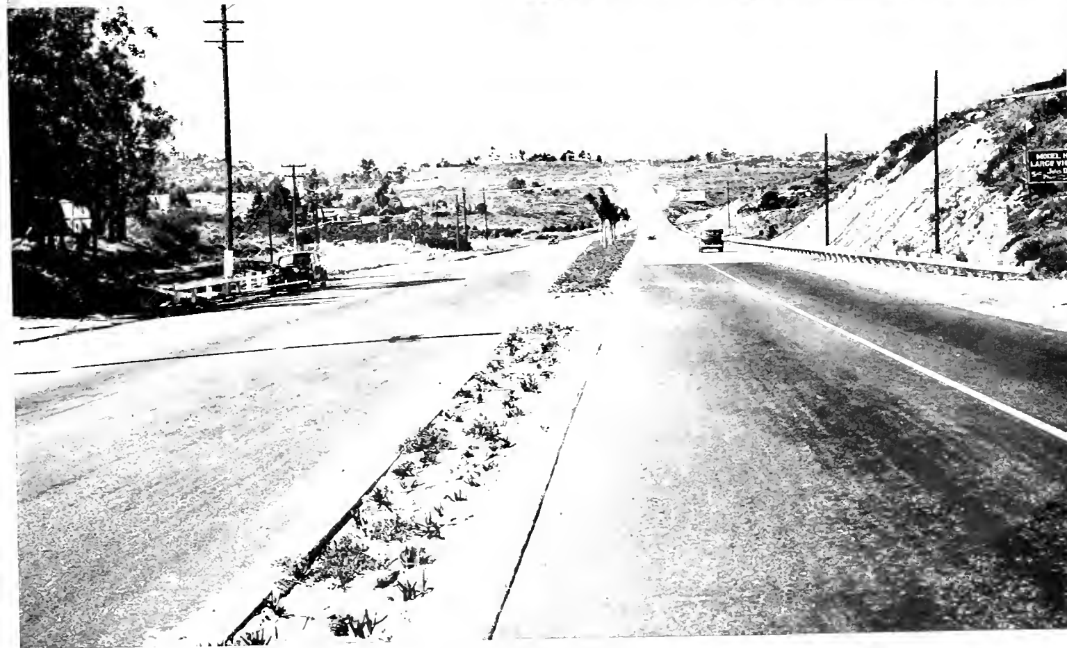
The four-lane divided highway cut-off recently completed in San Diego County between La Mesa and El Cajon includes practically all features of modern design such as grade separations, opposing traffic separations by reflectorized curbs, profile separations and channelization islands
